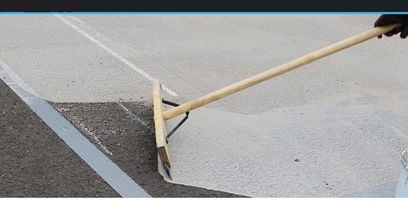
VersaFill W680 is a water based acrylic void filler which acts as a scratch coat, preparing bituminous substrates with a significant negative texture or uneven finish for the application of water based area coatings or DekorGrip resin bond coats. VersaFill W680 helps the final painted surface to have a more consistent and aesthetically pleasing finish and can also act as a barrier, preventing bitumen bleed on new asphalts. This is brilliant for areas such as electric car bays, loading bays etc.
