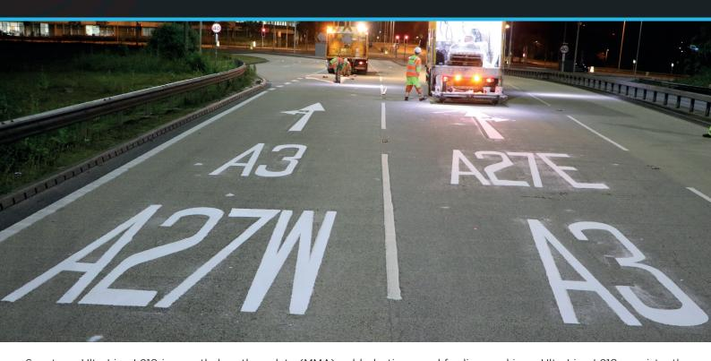
Spectrum UltraLine L210 is a methyl-methacrylate (MMA) cold plastic screed for line markings. UltraLine L210 consistently outperforms traditional thermoplastic as it is extremely hardwearing and has excellent adhesion to asphalt and concrete surfaces; this includes monoblocks and pavers. It can be applied by hand or using specialist application equipment for larger applications. UltraLine L210 is ideal for any transverse markings or high wear areas such as roundabouts and junctions.
