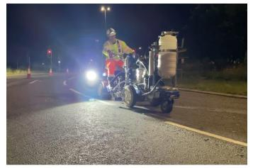
Not only the most environmentally friendly solution, cold applied electric line marking also offers the safest and most economical alternative to traditional hot works.
