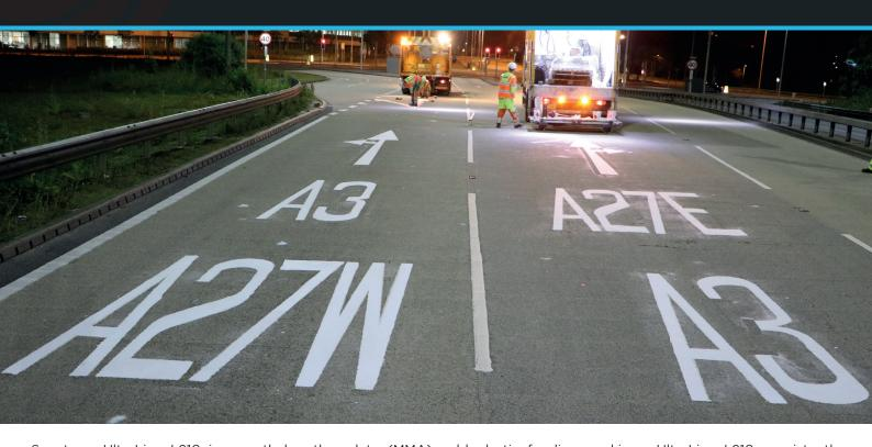
Spectrum UltraLine L210 is a methyl-methacrylate (MMA) cold plastic for line markings. UltraLine L210 consistently outperforms traditional thermoplastic as it is extremely hardwearing and has excellent adhesion to asphalt and concrete surfaces. It can be applied by hand or using specialist application equipment for larger applications. UltraLine L210 is ideal for any transverse markings or high wear areas such as roundabouts and junctions.
