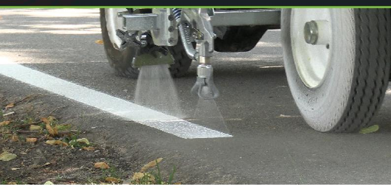
The Echostar 25 glass beads are high performance beads with a very high physical and chemical resistance and have excellent retroreflectivity due to a high quality manufacturing process ensuring over 80% bead roundness. Echostar 25 is a Type 2 bead which is designed to provide retro-reflectivity in both wet and dry conditions. The Echostar 25 beads are 1180-212µm which is suitable for use on line marking material applications of at least 590µm DFT. The beads are CE marked according to EN 1423.
