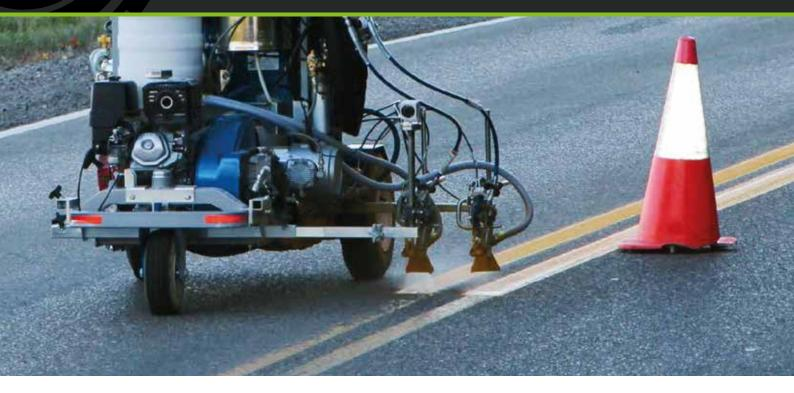
Basler Bascolin 2C CSP MP12 MMA Lining System is a solvent-free cold spray plastic for road marking based on reactive acrylic resin. Used for all forms of permanent surface markings on both asphalt and concrete surfaces for markings on highways, roads and other areas in the public and private sectors, as well as maintenance markings Type I and II. Airless spray application in a closed mixing system.
