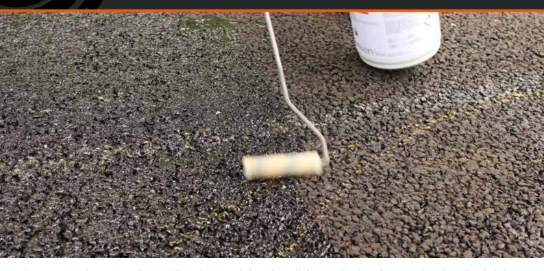
UltraNuvo is a clear primer designed for priming asphalt surfaces before application of MMA and PU-based anti-skid and slip-resistant coatings. It has a very short cure time, reaching full strength by the end of the cure time. This enables it to be used as a primer for new laid surfaces as any bitumen "bleed" is caught within the primer and prevented from migrating to the finishing treatment.
