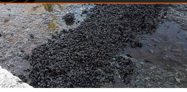
PatchMaster H576 is a high-performance cold patch asphalt mix for permanent utility reinstatement and repairing potholes or damaged surfaces on roadways, car parks, pathways and other asphalt surfaces. It has been proven to outlast the surrounding substrate, and can be used all year round in all-weather applications – wet or dry. PatchMaster H576 is supplied ready-to-use and requires no primer for quick fix applications.
