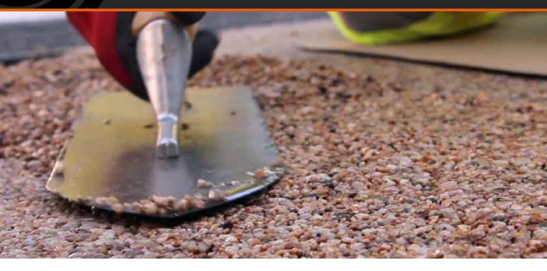
An encapsulated natural aggregate resin repair kit. Perfectly meets current demands for sustainable drainage (SUDS) whilst ensuring a stunning surface. For use in resin bound surface where an area needs to be reinstated or repaired. Matched to suit and naturally blends in with existing surface.
