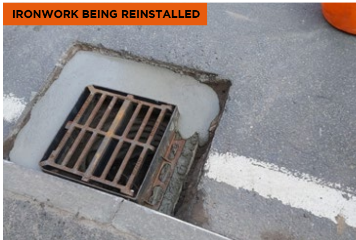
REINSTATING WITH HARDMASTER W615 & PERMAFYX L271
