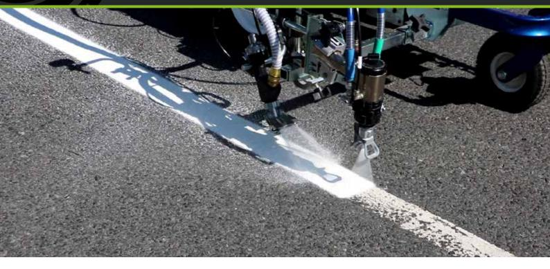
The Graco LineLazer 200MMA 1:1 MMA machine is a reliable walk-behind solution that delivers superior MMA 1:1 performance and guarantees ratio assurance in a compact and affordable package. This machine features an air-purge gun design which allows for the product to be mixed in the gun, lowering the risk of product drying in the hoses and eliminating build up of material at the tip.
