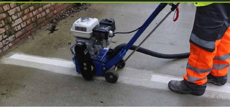
The Graco GrindLazer Standard DC87 G is a forward cutting drum scarifier which is ideal for basic surface preparation, repairs and line removal. It excels in smaller traffic marking removal jobs, trip hazard removal and for surface preparation before applying new traffic markings. The GrindLazer DC87 G can be linked up to a LazerVac system to reduce airborne silica dust.
