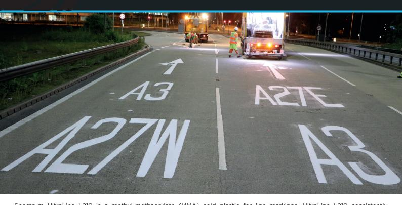
Spectrum UltraLine L210 is a methyl-methacrylate (MMA) cold plastic for line markings. UltraLine L210 consistently outperforms traditional thermoplastic as it is extremely hardwearing and has excellent adhesion to asphalt and concrete surfaces. It can be applied by hand or using specialist application equipment for larger applications.
