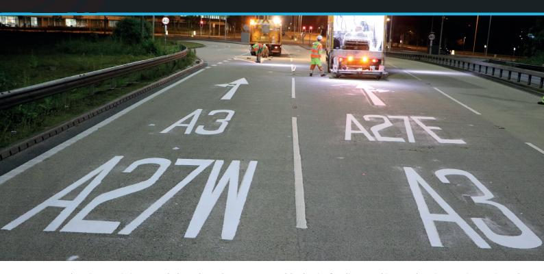
Spectrum UltraLine L210 is a methyl-methacrylate (MMA) cold plastic for line markings. UltraLine L210 consistently outperforms traditional thermoplastic as it is extremely hardwearing and has excellent adhesion to asphalt and concrete surfaces; this includes monoblocks and pavers. It can be applied by hand or using specialist application equipment for larger applications.
