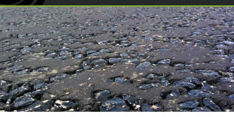
Pre-coated chippings are intended for use in hot rolled asphalt surfaces, increasing the skid resistance and durability of the road surface. These chippings have a 20mm aggregate size and up to 65+ PSV (polished stone value) for the black chippings.
