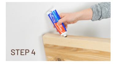
To create a permanent install, insert construction adhesive or silicone into each hole at the back of the shelf.
