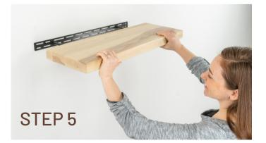
With even pressure, slide the shelf onto the front of the bracket. Allow the adhesive or silicone 8 hours to dry.
