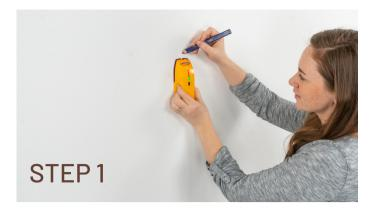
Use your stud finder to mark the locations of your studs. Be sure to mark the center of the studs (not the outer edges).
