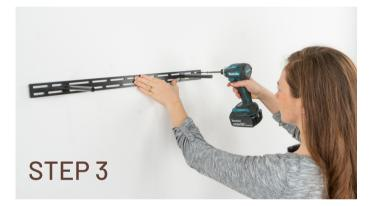
Hold the bracket firmly in place and drill a pair of screws into each stud location. (You will use a total of 6 screws).
