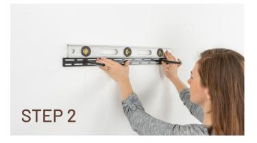
Place your bracket on the wall, aligning it with the stud locations you have marked. Adjust until level.
