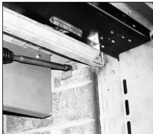
Step Four: Fix Side Liners in place using Liner Retainer Clips.
