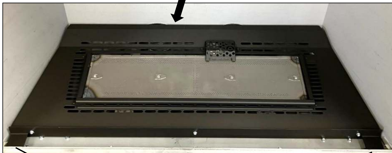
Tabs will rest against front ledge of firebox.
