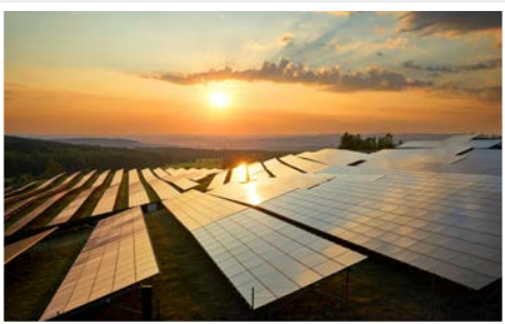
Compatible with BYO Solar Installs
