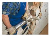
As a demolition tool, the DARDA HCS 6 **B** replaces the sledge hammer as a very efficient tool that will precisely break through brick walls up to 32 cm (12,6 inches) thick.
