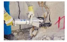
The HCS 6 J is able to crush concrete walls up to 15 cm (5,9 inches) thick (depending on compression strength of the concrete). A big advantage for breaking, separating walls, facade or reclamation concrete panels.
