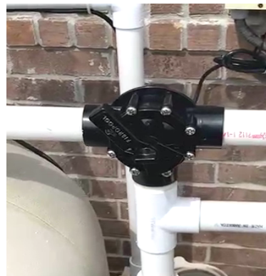
Throttled by pas valve, 50% open
