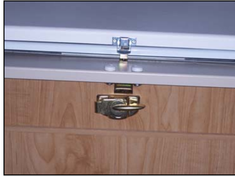
Retaining Latch Unlocked
