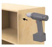
2. Drill holes using the 1/16" drill bit from the starter kit. NOTE: Drill no deeper than the red of the drill bit. (1/2" deep).
