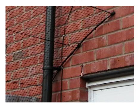
From that point you will require a bracket every two fence panels or four meters until you reach the end or a corner\* which will require a corner bracket. Cary on with a bracket every other fence post again to the end or another corner and so on until you have reached the end. If there is another wall as in the above photo eyelets can be used again to save a bracket.
