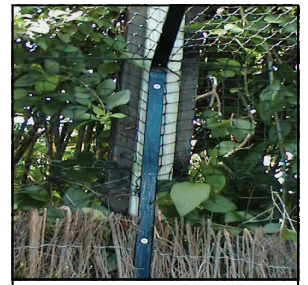
Bracket With Netting Behind
