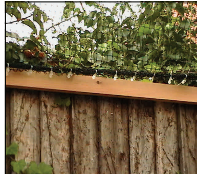
Cable Ties Trimmed
