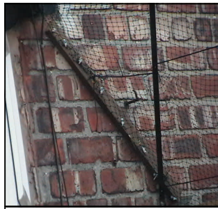
Batten attached to wall
