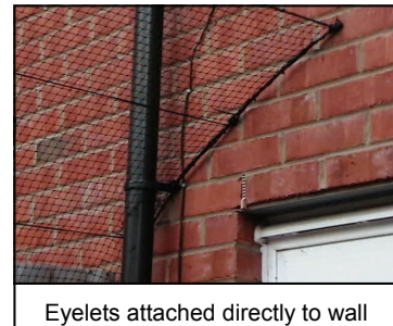
Eyelets attached directly to wall with cord strung between
