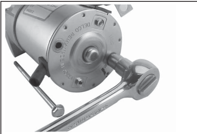
Figure 8-41. Removing Thru Bolts.
