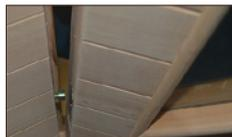
lift the panel with the male notch and insert it into the female notch of the other panel. press down to lock.
