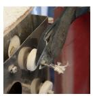
Cut the element pigtail between the porcelain insulator and the connector.
