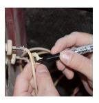
3. Label each feeder wire with a piece of masking tape and a number starting at the top. Taking a picture can also help when you are reinstalling wires.
