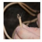
21. If you stripped 3/4" of insulation from a feeder wire fold over the exposed silver wire to make it thicker and improve the fit in the connector.
