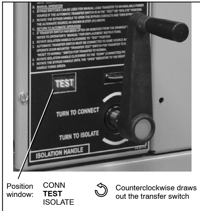
Figure 7-15 Isolation Handle Turned to TEST
