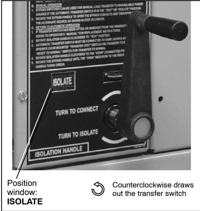
Figure 7-17 Isolation Handle Turned to ISOLATE.
