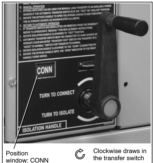
Figure 7-24 Isolation Handle Turned to CONN
