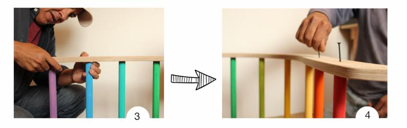
Place the arch on a flat level surface to make sure the arch is level and then tighten the screws. Press firmly. In case the arch is not level, loosen the screws and re-tighten as needed.
