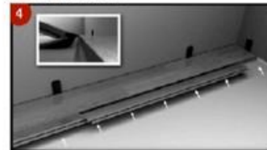
STEP 4: Raise 2 pieces of floor at an angle of around 30. Make sure that the lock on the short side is not disengaged.
