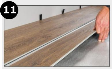
DISASSEMBLING THE LONG SIDE Lift up the entire row in the same angle as you did during installation, then slide the rows apart.
