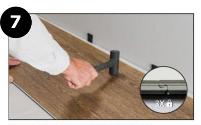
ENGAGE 3RD PLANK ON SHORT SIDE (Part II) Using a soft rubber mallet slightly tap the joints on the short side to secure. This ensures 3x locking.
