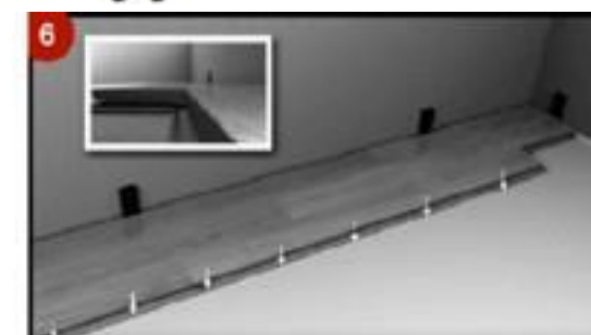
STEP 6: Make sure that the long side and short side tongue into the groove, and then drop down 2 pieces floor
