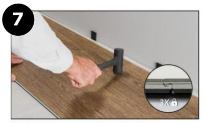
ENGAGE 3RD PLANK ON SHORT SIDE (Part II) Using a soft rubber mallet slightly tap the joints on the short side to secure. This ensures 3x locking.
