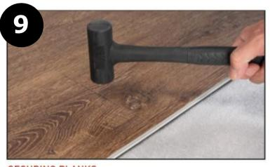
SECURING PLANKS As you go, don't forget to use a soft rubber mallet on the short sides to secure the locking.
