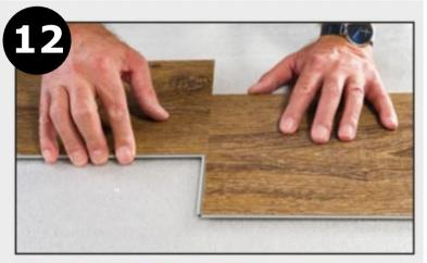
DISASSEMBLING THE SHORT SIDE Disassemble the row by sliding apart the planks on the short side.
