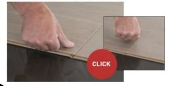
**DISENGAGE** - short side To disengage on the short side, softly slide the planks in opposite directions.
