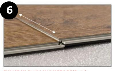
ENGAGE 3RD PLANK ON SHORT SIDE (Part I) Using the drop-lock one piece drop-lock system, drop the short side of plank 3 onto the short side of plank 1.
