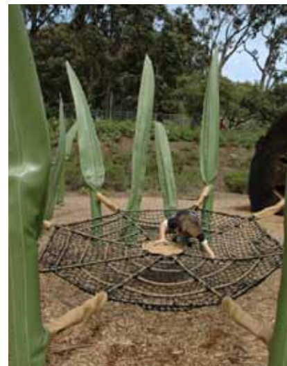
Netform spider web net anchored to steel columns with decorative coverings.
