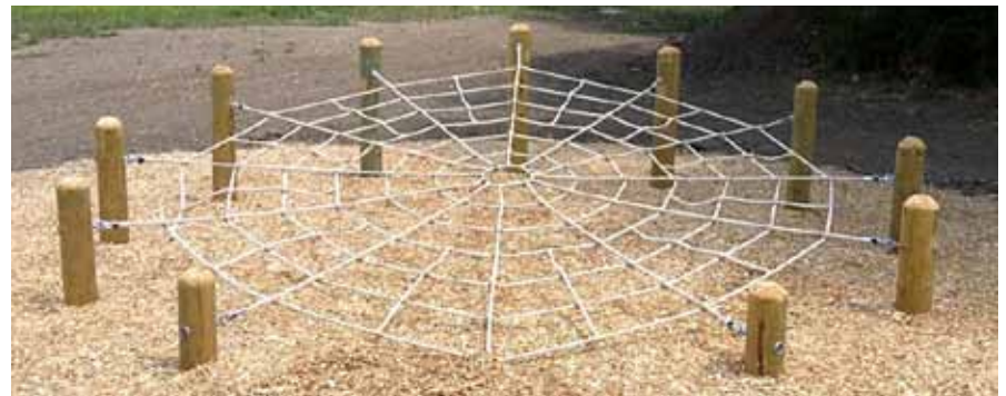
Rope spider web net anchored to wooden bollards.
