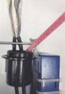
**12.** Dispense sealant. Follow instructions with closure sealant 10B. fill sealant to 10mm from top of port.
