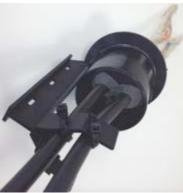
**11.** Seal cables to base of closure using putty to create a dam to prevent sealant from leaking.
