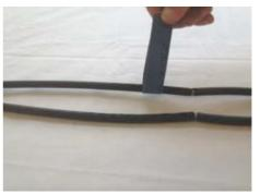
2. Critically important to abrade cable for a distance of 150mm below the stripping port using the abrading tape provided. Clean again with PF Wet & Dry wipes after abrading. Clean and dry the inside of the closure base with the PF Wet and Dry wipes to remove grease and other residues
