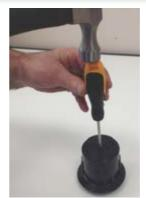
Choose the size of the cable entry knockouts. Use appropriate size screw driver to knock out the hole. Ensure to turn the screw river to remove any sharp edges on the hole that has been punched.
