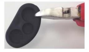
**3.** Determine the cable layout and cut D shaped grommet accordingly, this adaptor allows a maximum of 3 cables. Refer to cable layout guide.
