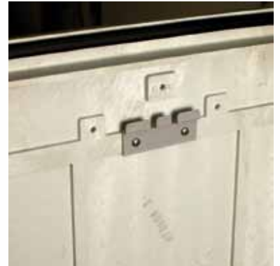
2. Fitting the fixing bracket to the cabinet door. Secured using 2 self tapping screws.
