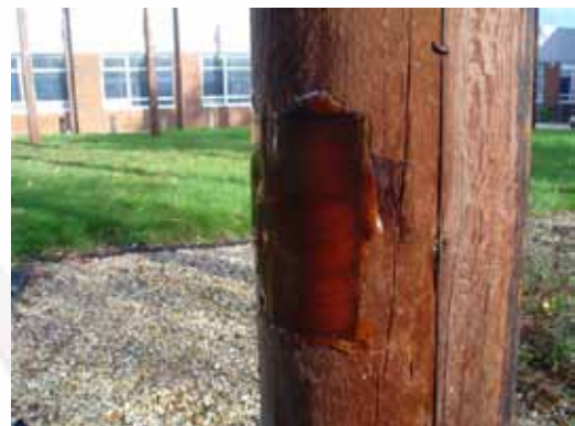
Finished resin repair area
