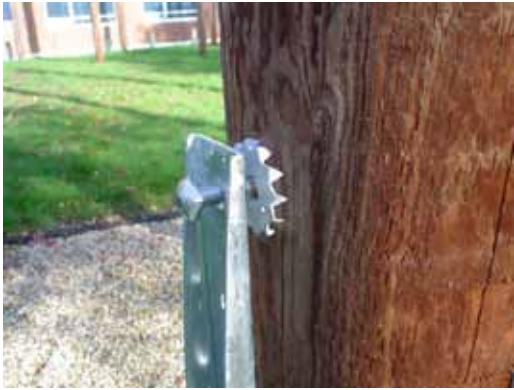
First bolt, with Toothplate connector, ready for tightening
