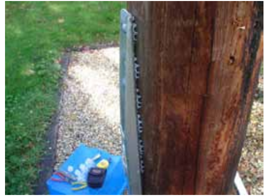
Strap fully bolted
