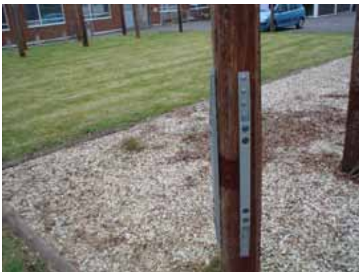
Complete job, with both straps fitted, either side of damaged/resin repaired area NB –these photos show the old style repair strap
