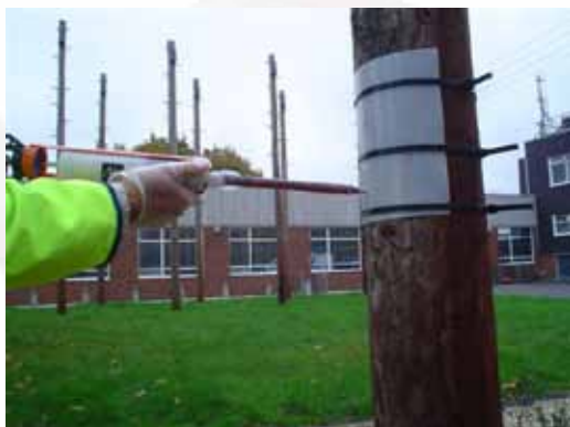
Applying the resin. Note hole lowermost
