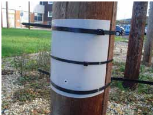
Damaged area, with shield fixed in place
