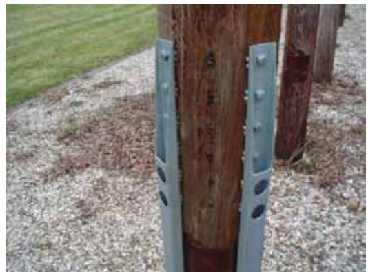
Complete job, with both straps fitted, either side of damaged/resin repaired area NB –these photos show the old style repair strap
