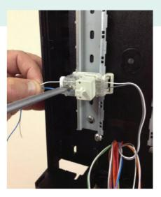
Moving to the drop wire side screw 8 Moving to the drop who ever connection. Cut the single pair wires equally and then insert fully into the port entry holes. Screw down the housing until you come to a stop. No need to over tighten.
