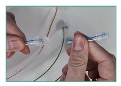
The old connector is cut away without any break in service.
