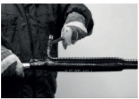
2. Using a suitable tool pull the stainless steel rail away from the wraparound guides as shown. Remove the entire rail from the sleeve.
