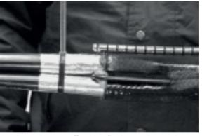
16. Press branch-off cables firmly together and secure with cable tie.
