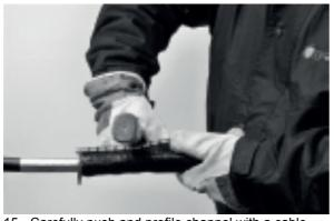
15. Carefully push and profile channel with a cable dressing tool to follow the form of the transition area.
