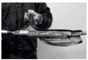
Ensure to use safety glasses and protective gloves. Re-heat the closure. Using a suitable tool and working from one end gradually remove the wraparound sleeve.
