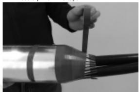
Tape the canister ends, start from the metal canister, down to the cable ensuring a 50% overlap. Do not tape more 5mm onto the cable.
