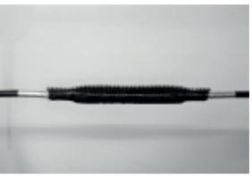
18. When all temperature paint has been converted to black over the closure, two separate lines should be visible in the slots of the channel. If at any point the two white lines are not visible, then reheat the closure at that point until the lines appear. After installation, allow the heat shrink sleeve to be completely cool normally 45 minutes is required.
