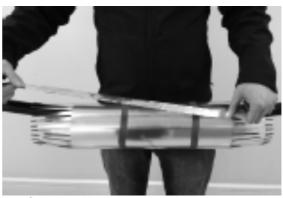
Center and Install metal canister over the joint bundle. Seal canister seam with adhesive aluminium tape.
