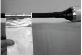
Wrap aluminium foil onto cable as shown. Start at the inner mark and apply away from the canister.
