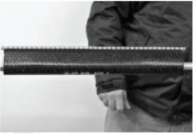
Push the flexible stainless rails over the channels. Slide the retaining clip into position. The clip should be centrally positioned to retain each rail equally.
