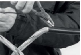
If a grounded wire is required, use suitable tool to cut a tab in the cable jacket over a length of 25mm. And a width of 15mm.
