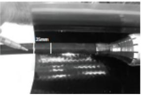
Center the sleeves over the metal canister and mark the sleeve ends on the cables. Then add a second mark a thumb width (25mm) nearer the liner.
