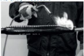
Re-heat the wraparound sleeve starting from one end and working along the rail area to the other end of the sleeve.
