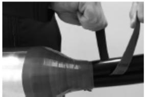
Abrade the cables circumferentially over a minimum of 20cm and clean once more.
