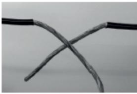
Remove cable shield jackets and complete the joint. Finished joint opening length should be length "L" as in table (see last page "Normal Sheath Opening L"
