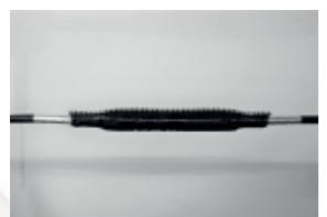
17. Adhesive must flow from the ends of a sleeve when properly shrunk. If the adhesive does not flow out of the sleeve, re-heat again until the adhesive appears.
