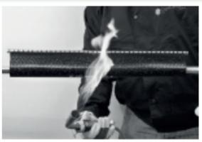
14. Begin the shrinking process from the bottom, centre section. Continue to shrink that area until the indicating paint has changed color. When the paint has completely changed to black gradually move the flame towards the channel area. Move to one end of the sleeve and shrink as before. Shrink toward the branch end first.
