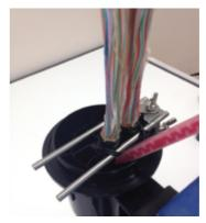
**12.** Dispense sealant. Follow instructions with closure sealant 10B. Fill sealant to 10mm from top of port.
