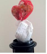
14. Remove 100g silica gel from the bag. Sign and date label. Place 100g silica gel into mesh bag and tie to conductor bundle. Replace Silica gel each time the closure is opened. Silica gel changes from yellow to green to indicate it is to be replaced.
