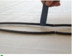
2. Critically important to abrade cable for a distance of 150mm below the stripping point using the abrading tape provided. Clean again with PF Wet & Dry wipes after abrading. Clean and dry the inside of the closure base with the P/F wet/dry wipes provided to remove grease and other residues.
