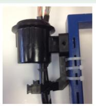
**9.** Secure the closure to the pit guard using the re-useable large cable ties provided.
