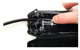
Insert cable ensuring a minimum of 15mm of sheath is protruding into the gel.
