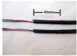
Prepare cable using current work practices. For hard jacket cables, remove 45mm of outside sheathing in order to fit into the entry slot of the closure.
