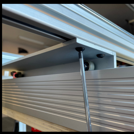
STEP 3-3: Tighten Rear Bracket
