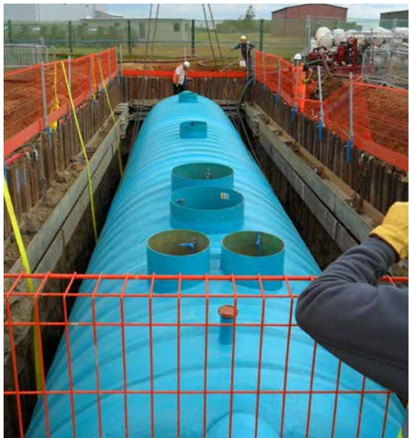
SPEL Separator being installed at an RAF base.
