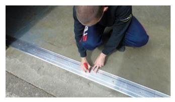
Return the threshold seal to an upright position and lay it into position across the opening. Using a marker pen/pencil, mark where to drill the holes in the concrete.
