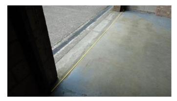
Determine whether the threshold is to be fitted between the door tracks, or mitred around the tracks.
