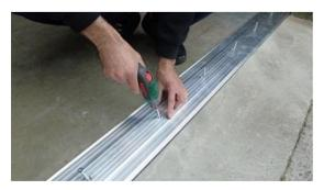
Apply pressure to the threshold seal with your foot. Using an electric screwdriver, tighten the screws into place making sure they are flush but do not overtighten.
