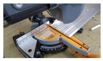
(a) Mark and cut the threshold to size to sit in between the door tracks. (b) If fitting the threshold seal around the door tracks, measure the distance between the wall and the back edge of the threshold seal and cut the end sections to this length. Using a mitre saw, cut the threshold seal sections accordingly.
