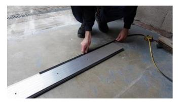
Turn the threshold section(s) upside down and insert the bottom seals into the grooves at either end of the threshold.
