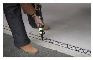
In the case of the floor being uneven, lay a bed of adhesive underneath where the threshold seal is to be fitted to ensure a watertight seal. With the threshold seal in position, mark along the front and back edge of the seal with a marker pen/pencil. Remove the threshold seal and mark a line approx 10mm inside the existing lines, followed by a zig zag line in the middle of them. Apply adhesive & sealant following the pencil lines created.
