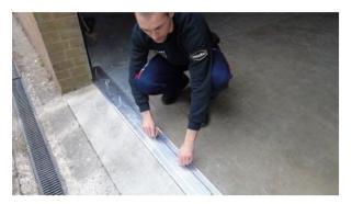
Place the threshold seal back into position. Insert all of the screws in their respective holes and hand tighten each of them. Then ensure that all screws fit snugly.
