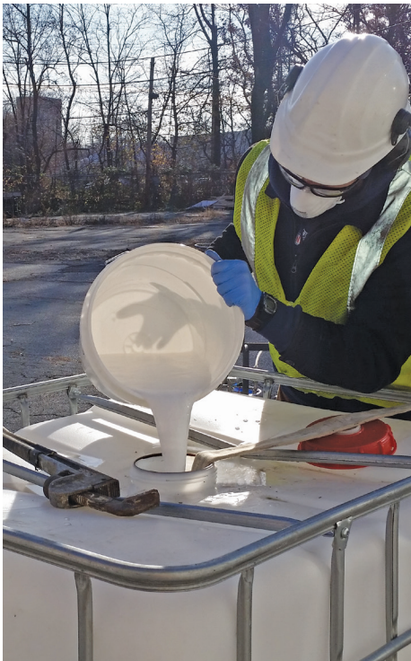
Field technician preparing anaerobic injection water with KB-1 ® Primer slurry
