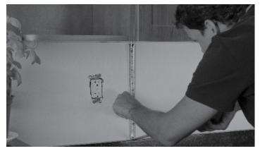
B. Place a sheet of mosaic on your counter, cut to appropriate size and test on the wall without peeling the back.
