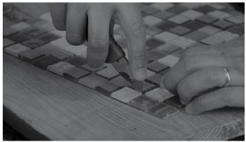
C. Choose an alignment reference (horizontal and vertical) that is level (e.g., the corner of a wall, the top of the counter). Don't forget to check the top, bottom and sides of the tile to make sure it lines up.
