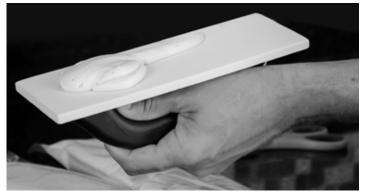
bottom to top. Bring the float back across the mosaic in the opposite direction applying additional pressure. Check to see if the joints are completely filled with grout and all excess grout is removed from the tile. Repeat until complete the entire backsplash.
