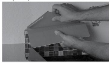
B. Begin the installation from left to right completing the bottom row first. After installing your first row you can begin installing the top row. Take your time and make sure you align the grout joints before you apply pressure. Once you are happy with how your grout joints are lined up use your grout float to apply even more pressure to assure good adhesion to the wall.
