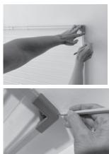
Place the finished frame on the selected area of the ceiling and mark the 4 corners.
