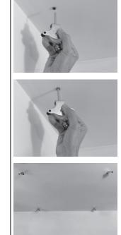
Using the drill (8mm drill bit), drill a hole (50mm deep) in each mark. Insert the DOWEL FOR PULLEYS "I" and then, in
