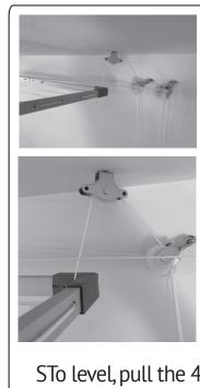
Hang the frame by threading the rope from each corner into the corresponding pulley on the ceiling. Take the ropes and bring them to the DOUBLE PULLEYS FOR WALL "J"; spread them out so that they do not cross each other.
