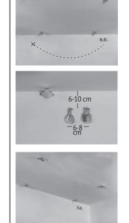
Place the 2 DOUBLE PULLEYS FOR WALL "J" on one side of the frame on the wall at a distance of 6-10 cm from the ceiling and 6-8 cm from each other. Remember to use the DOWELS FOR PULLEY "I" if necessary.
