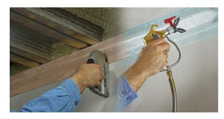
extension of a 1-3/4 in (44 mm) joint. It also allows extension in joint movement for Class 1 (500 cycles at 1 cycle per minute (cpm)), Class II (500 cycles at 10 cpm) and Class III (100 cycles at 30 cpm) joint applications as required by the applicable building code.
